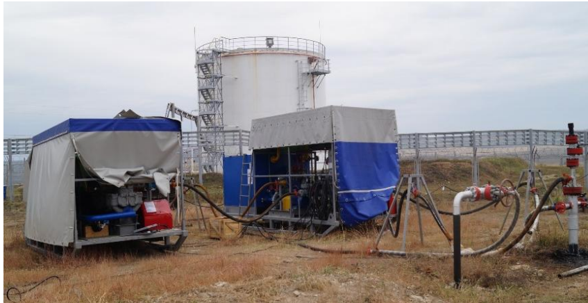
Fig. 2. Field tests of MPU
